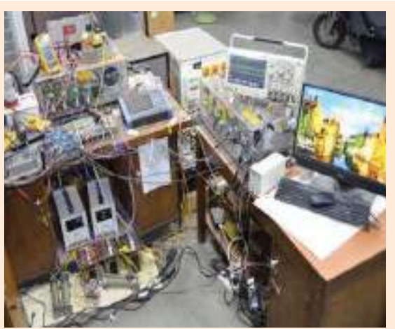
EV Battery Charging Setup facility from Grid
